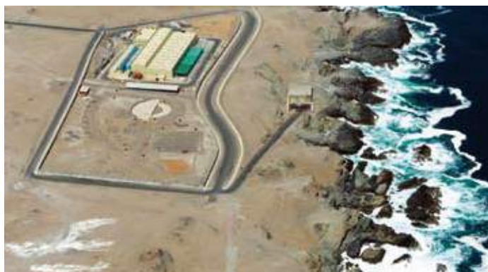
Desalination plant at ADASA
