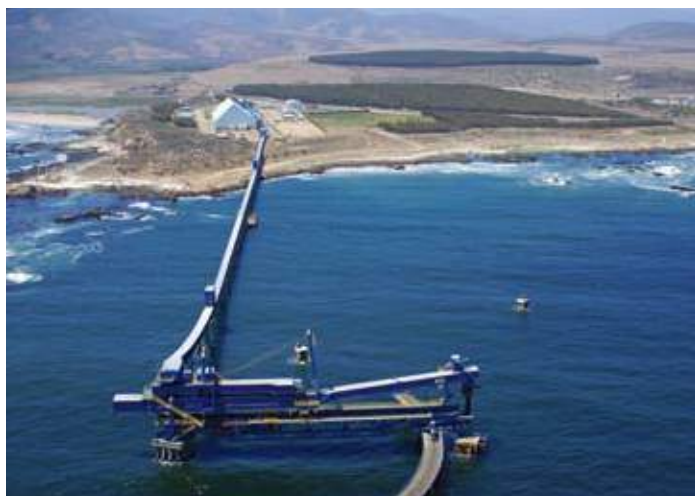
Los Pelambres port facility at Punta Chungo
