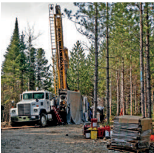
Drilling work in progress at the Twin Metals' project in Minnesota.
